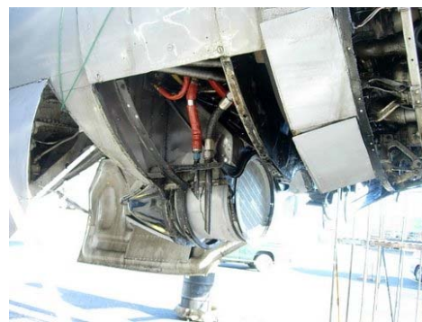
The new oil cooler for the #2 engine. On this inspection, all four oil coolers were removed for overhaul and reinstalled. This was a big job and took a lot of time
